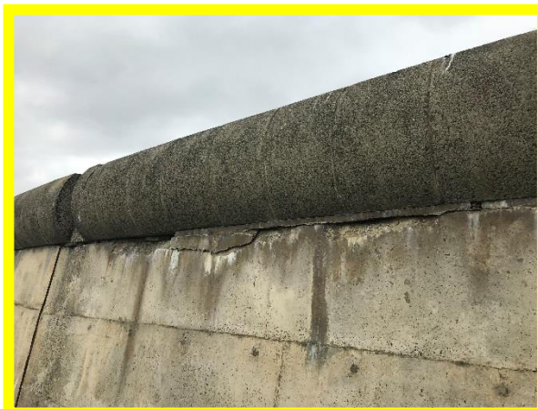
Loss / wash-out of mortar beneath coping. Local abrasion (/0601C01)
