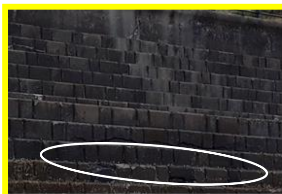
Longitudinal crack in blockwall wall (/1201C08)
