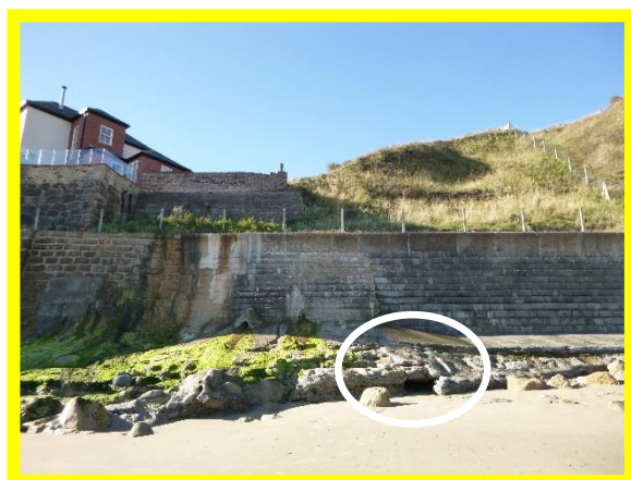
Private sea wall in fair condition. Large void visible in wall apron. (/1402C02)
