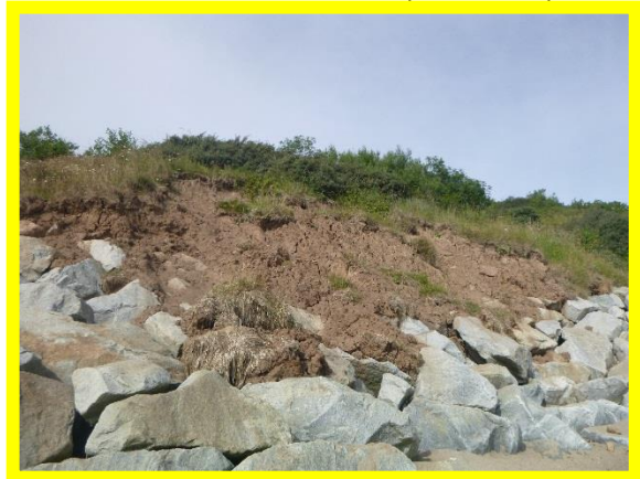
Slumping of cliffs behind rock armour (/1003C07)
