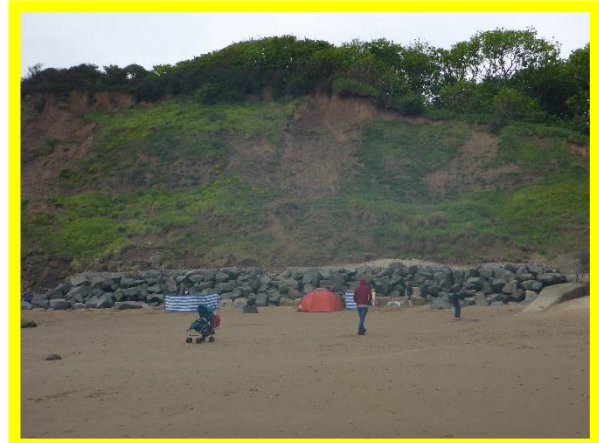
Rock revetment at southern end of Filey Sea Wall (/1602C02) – note active coastal slopes to rear
