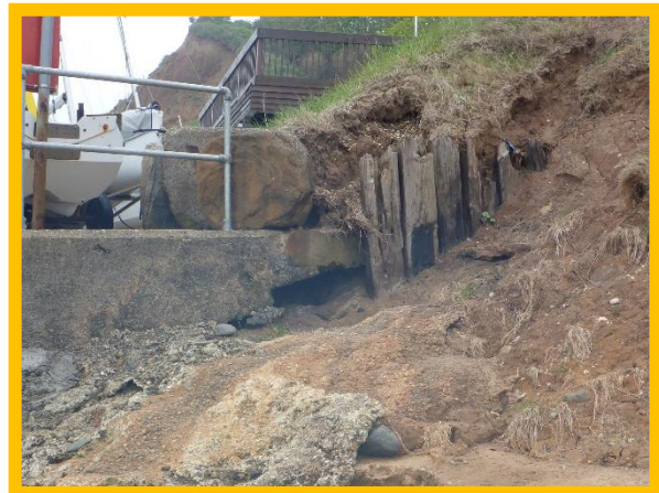
Scour hole at northern end of promenade (/1601C03)
