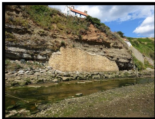
North bank: Works completed in 2013 to repair collapsed cliff (no asset ref)
