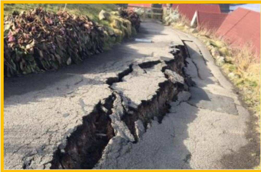
MU22/4 Large cracks in footpath above retaining wall failure
