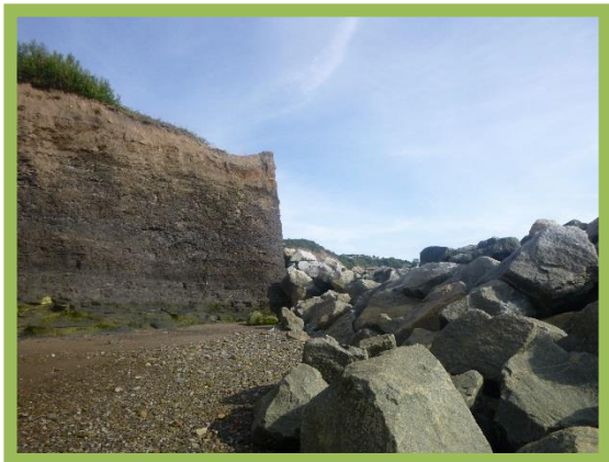
Rock revetment protruding beyond undefended cliffs (/1003C01)
