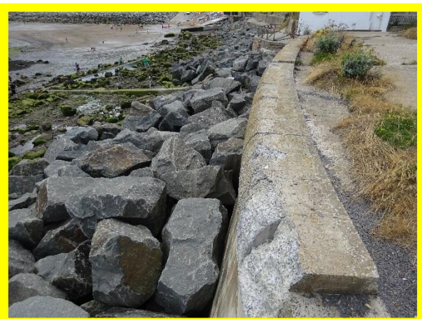
Abrasion and cracking of concrete coping (/0601C01)
