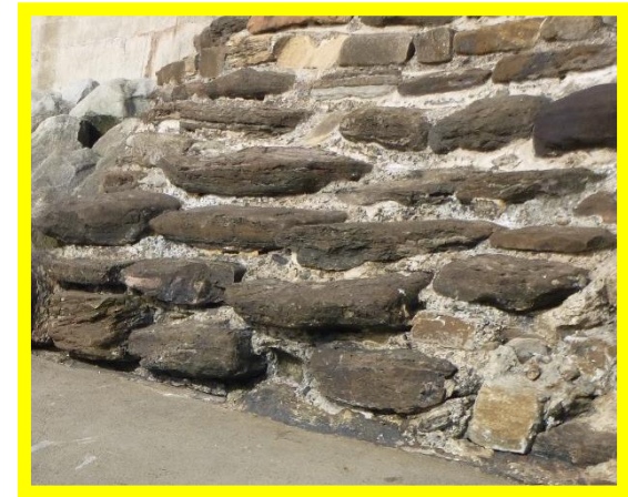
Typical defects (gaps) on blockwork wall (/1003C06)
