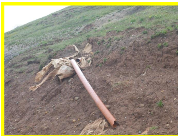
MU11/1 Evidence of slumping and broken pipe in the lower coastal slopes (Locally Active)
