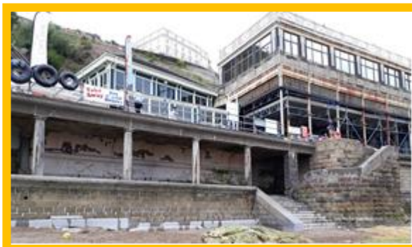
Previous repairs (Dec 2013) at the open colonnade remain effective, but extensive open joints remain in lower wall (/1302C01)
