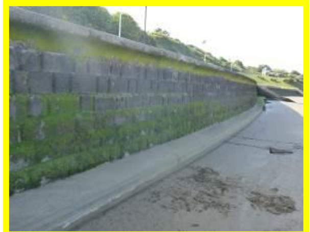
Fair condition seawall with recent repairs to toe apron (/1201C24)
