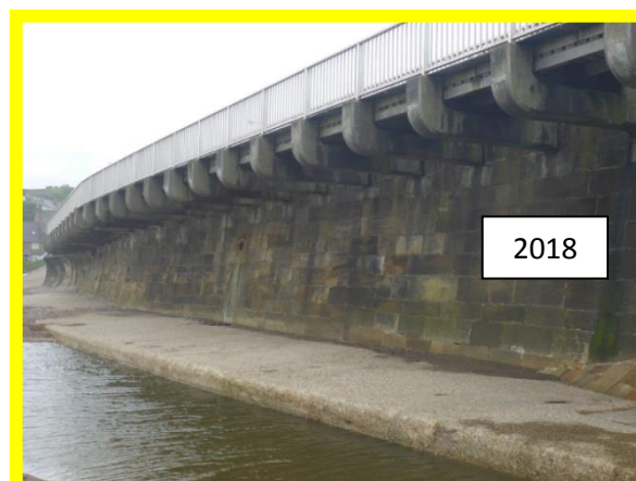
Masonry blockwork sea wall with cantilevered footway (D0702C04)
