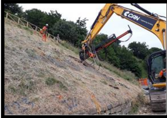
MU22/2 Soil nail installation on coastal slopes near the Spa
