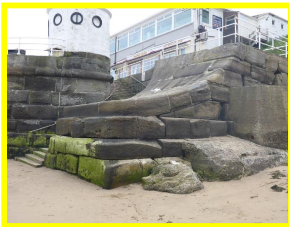
Open joints in wing wall to access steps (\D0802C12)
