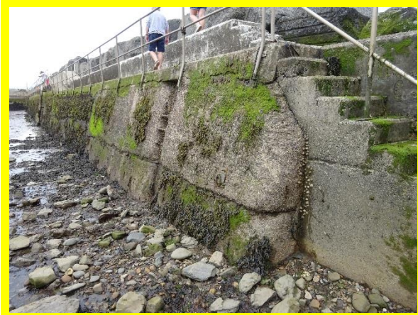
Local abrasion, cracking and spalling inside face of South Breakwater (/0403C03)
