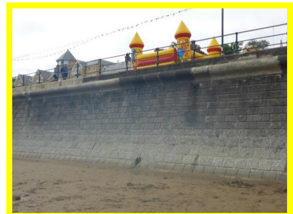
Previous repairs to coping and wave return feature (/1602C08)
