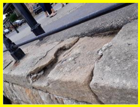
One of the worst areas of abrasion at top of wall (/1301C25)
