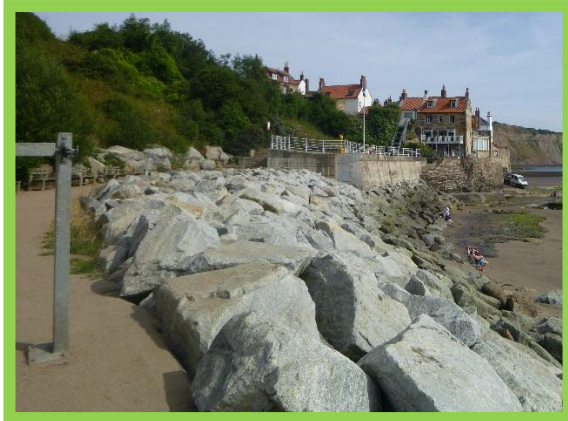
Rock revetment and slipway remain in good condition (/1003C09)
