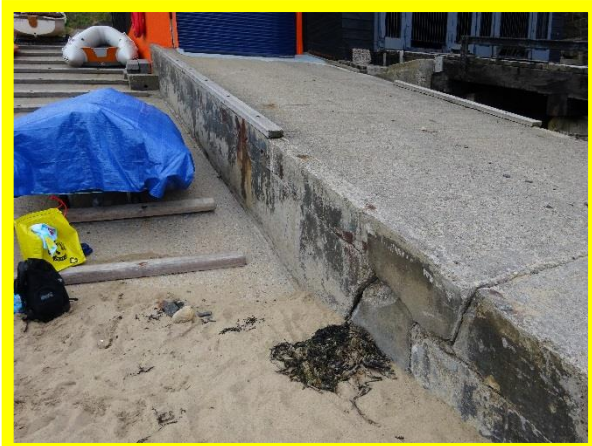
Open joints / cracks in Runswick Rescue slipway (/1003C04)
