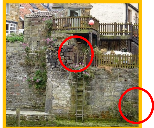
Open joints and loose masonry blocks locally (/0402C04)
