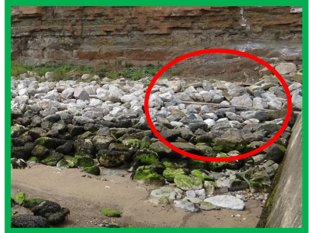
Lower crest level at northern extent of rock revetment (/0402C02)
