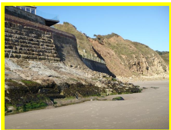
Private sea wall in fair overall condition but with the toe apron subject to ad hoc repairs and localised undermining (/1402C05)
