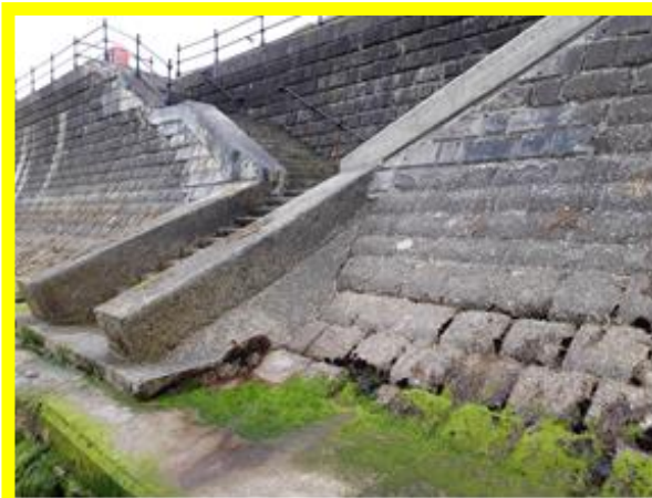
Previous repairs to wing-wall (/1201C07)
