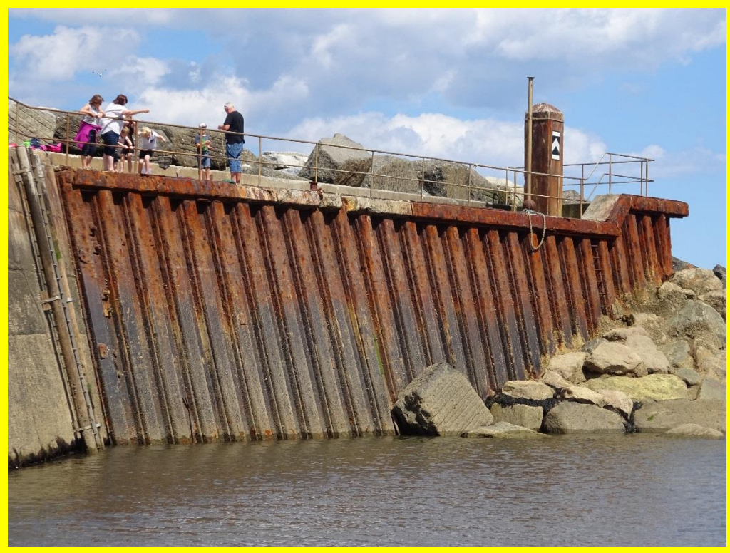
Corroded steel sheet piling on inner-face of North Breakwater (/0402C01)
