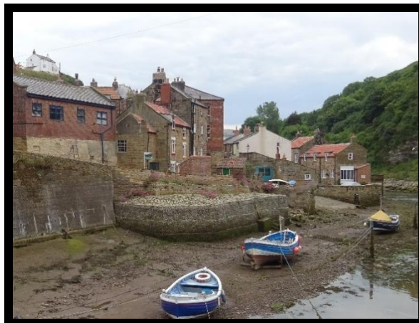
South bank: Stone-filled gabion baskets constructed in 2013 to repair collapsed wall (no asset ref)
