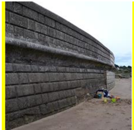
Area of heavy abrasion damage to promontory wall (/1201C04)
