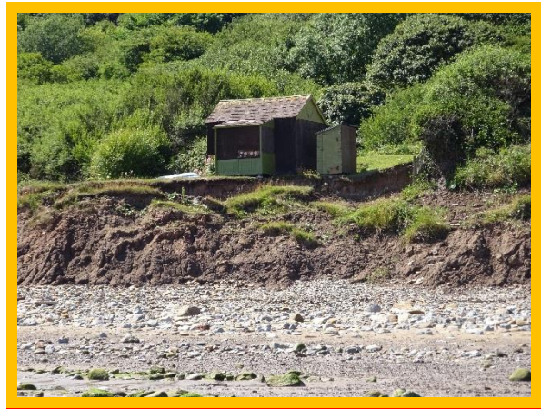
Slips are threatening the stability of timber buildings/sheds (use unknown) MU7/3N Partly Active in July 2018.
