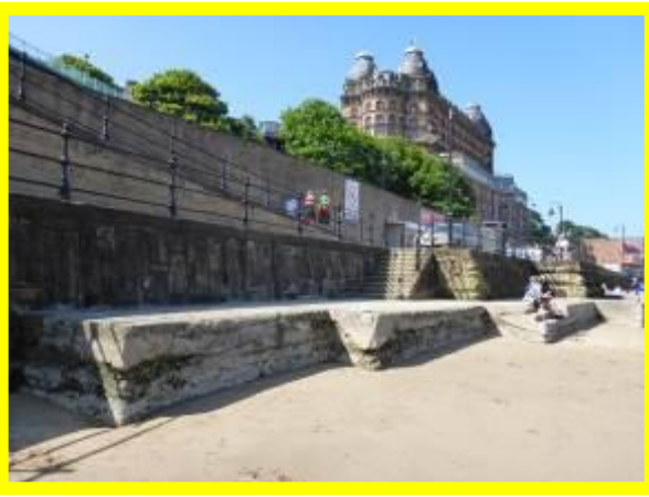
Abrasion of toe apron south of previous repairs (/1301C09)
