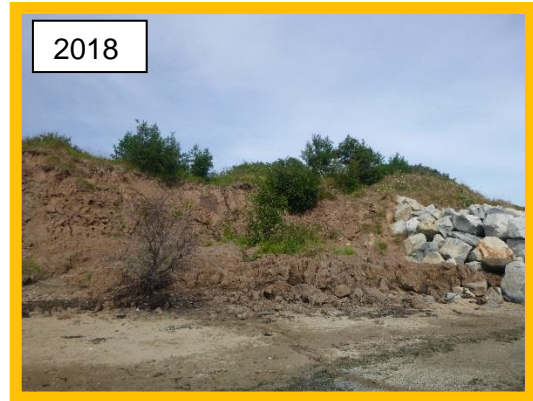
Slumped toe of till cliffs adjacent revetment. MU17/2 (Partly Active)
