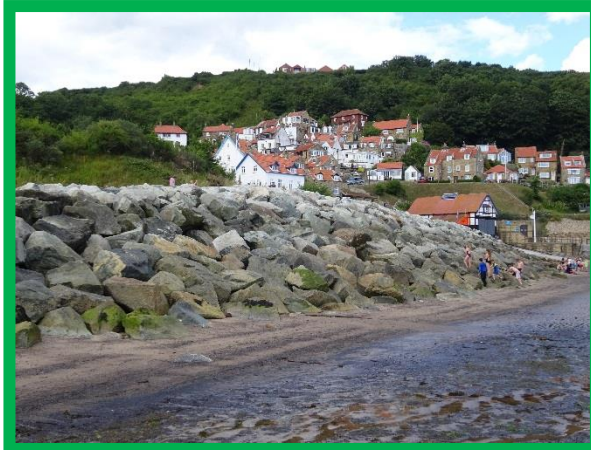
Rock armour revetment (/0602C01)
