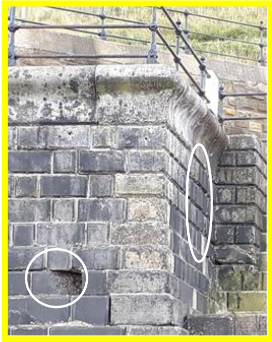
Southern end of wall with partially missing block and cracks on return (/1202C23)
