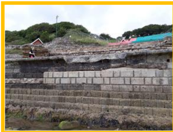
Overall fair condition of low stone wall with spalling to splash beam (/1302C02)
