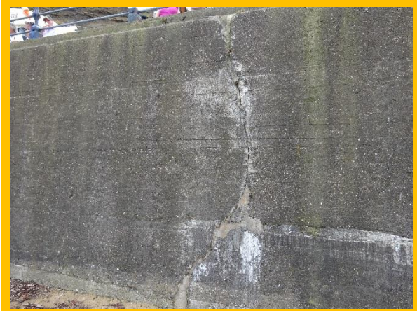
Previous repair to vertical crack washed out (/0403C01)
