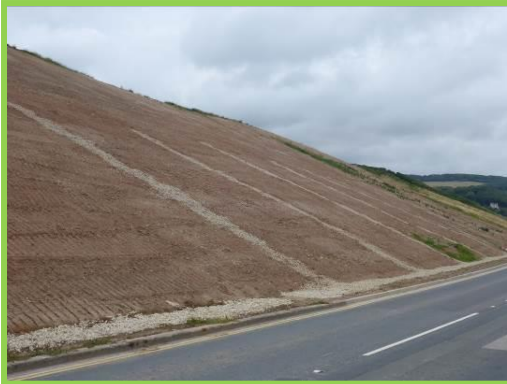
MU9/3 Coastal slopes to rear of new sea defences generally in an inactive state following capital works involving re-grading, drainage and seeding as part of the Sandsend Road Coast Protection & Slope Stabilisation Scheme
