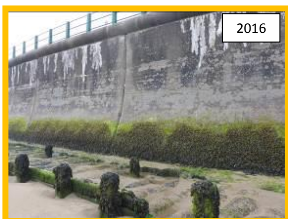
Poor condition sea wall (D0702C01)
