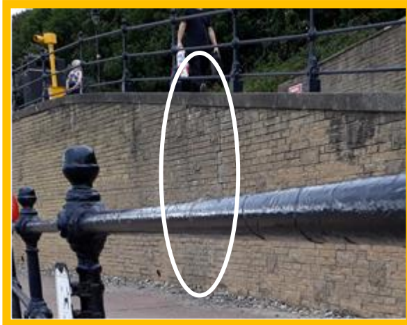
Vertical crack in wall above access ramp (/1301C10)
