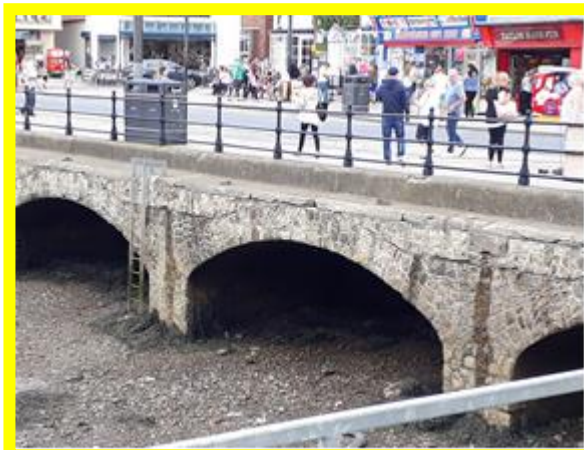
Some Cracking and missing joints to top of capping to wall south of roundabout opposite arcade. (/1301C05)
