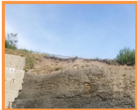
Erosion of cliffs immediately adjacent to large northern end of large sea wall (/1003C03)
