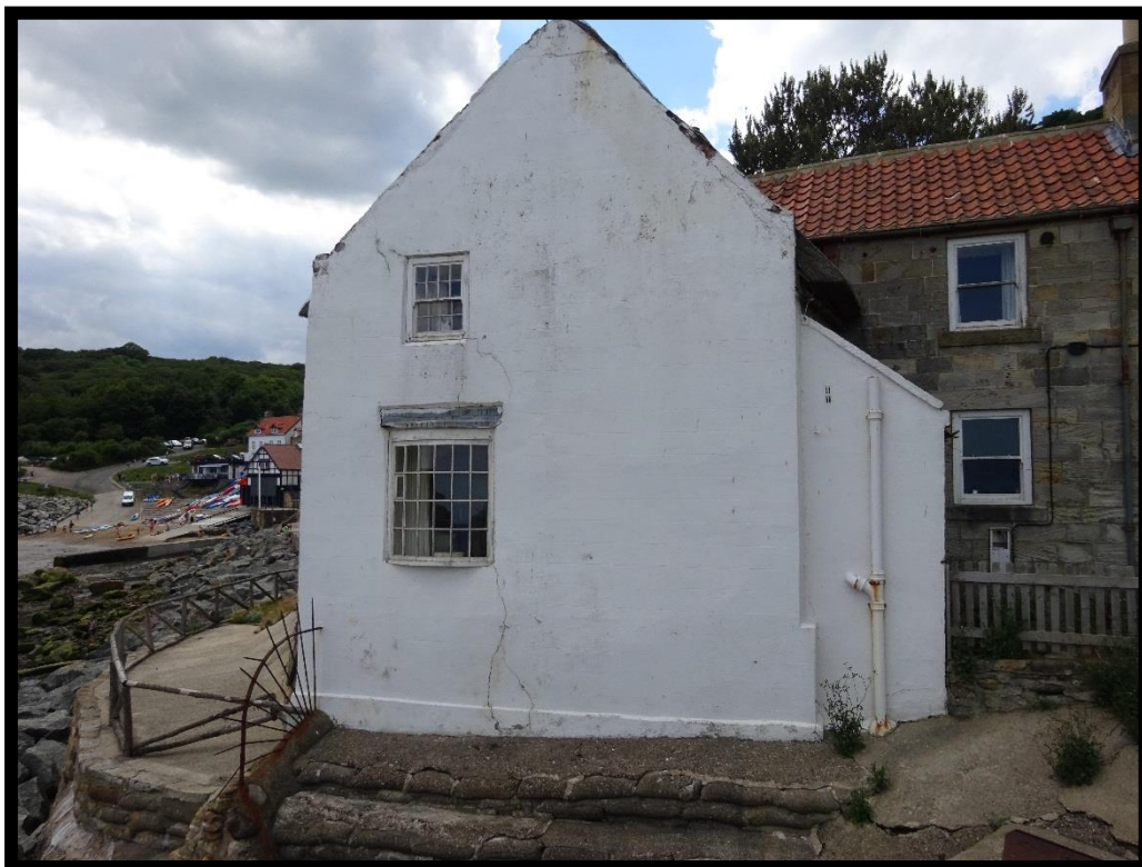
Cracks in gable end of Thatched Cottage
