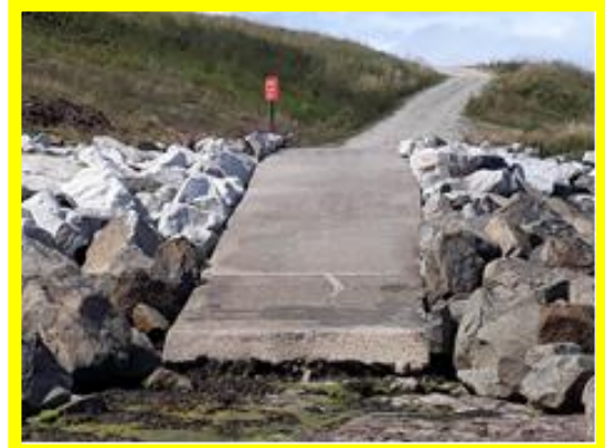
Vertical drop and crack in concrete at end of access ramp at south end of revetment (/1304C01)
