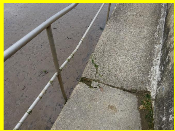
Local damage. Cracking and loose concrete to crest of South Breakwater. (/0403C03)
