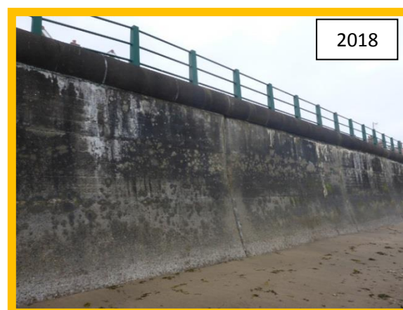
Poor condition sea wall (D0702C01)
