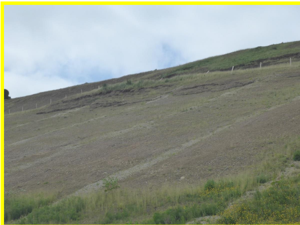
MU9/3 One area of locally active cliffs in the recently stabilized area. This shallow slip is to be remediated imminently.
