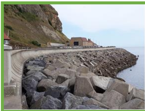
Accropode revetment with concrete toe piles, rock crest and wave return wall (/1202C02)
