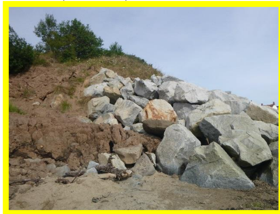
Outflanking of rock armour (/1003C07)
