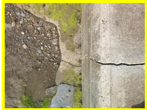
Typical defects (cracking) on toe apron (/1003C06)
