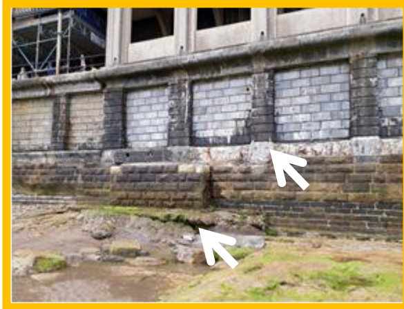
Spalling to the lower splash beam at closed colonnade section and undercutting at toe (/1301C29)
