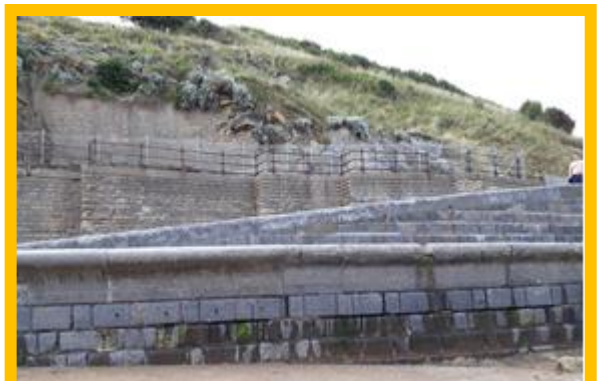
Seawall in overall poor condition Cracks to bastion throughout. Missing pointing / open joints and damaged parts of upper and lower capping beam. Mortar missing between blockwork in lower wall. Corroded handrail with missing sections. Upper prom has been fenced off. Full height cracks through uppermost wall. (/1304C02)
