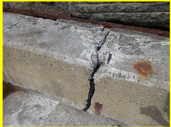
Crack in deck and crest wall of North Breakwater (/0402C01)
