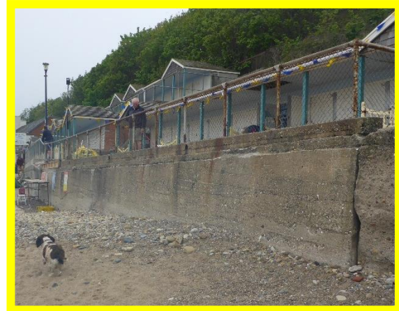
Longitudinal cracks in rear wall, open joint (/1602C01)
