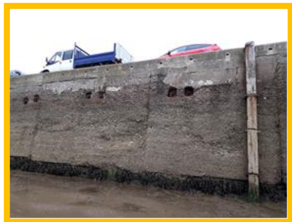
Spalling and loss of render in south face of West Pier wall (/1301C07)
