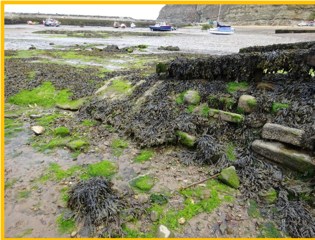
Open joints, loose masonry, missing blocks and undermining to North face of slipway (/0402C22)
