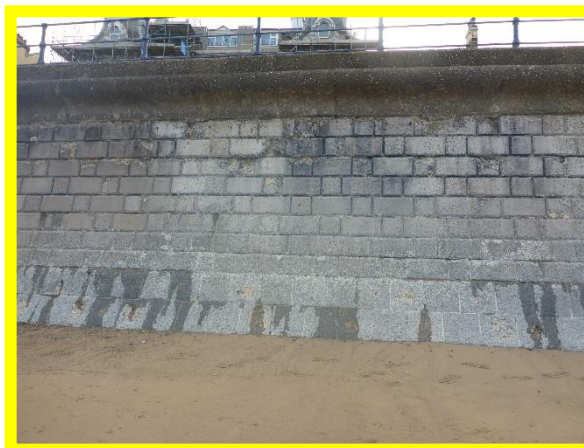
Abrasion damage, several leaking joints (/1602C03)
