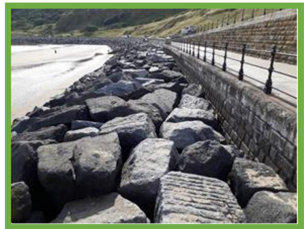
Rock revetment fronting seawall (/1202C01)
