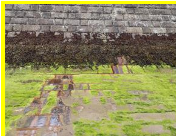
Leak through previous crack repair to seawall (/1201C07)
