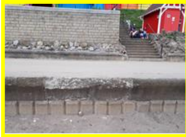
Abrasion of capping beam on front wall (/1201C05)
