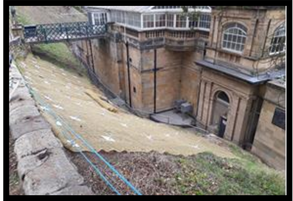
MU22/2 Soil nail and slope mesh installation behind main Spa building
