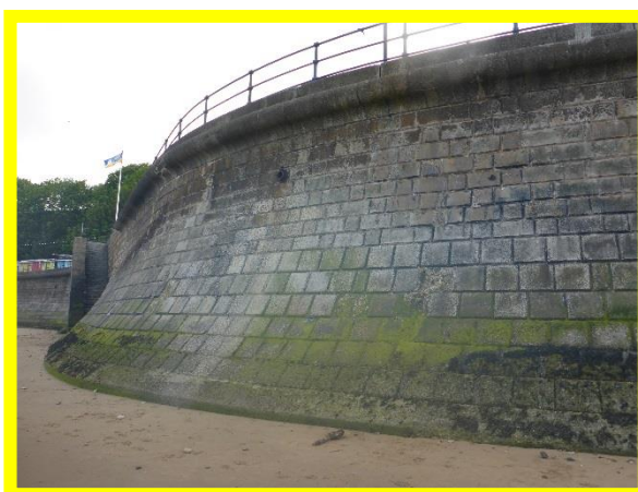
Royal Parade seawall in fair condition, some blockwork abrasion and open joints (/1602C04)
