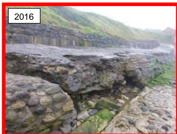
Undercutting at toe leading to voiding behind and break-up of deck (/1402C04)
