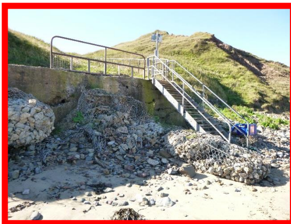
Failed gabion baskets at surf shop car park beach access (no asset reference)
