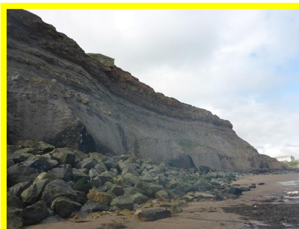
Rock armour protection to toe of Abbey Cliff (\803C06)
