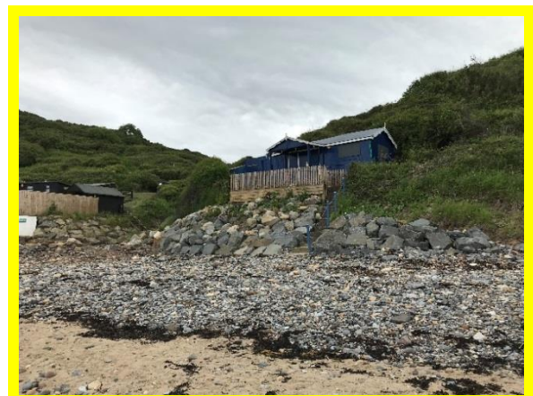
Rock armour slope protection at southern extent of MU7/3S , Locally Active in July 2018.
