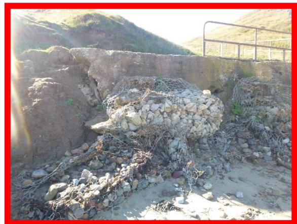
Failed gabion baskets at surf shop car park beach access (no asset reference)
