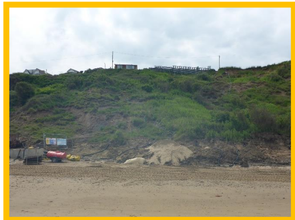
Works to install inclined drains at the toe of till cliffs at Flat Cliffs. MU29/AQ Partly Active in June 2018
