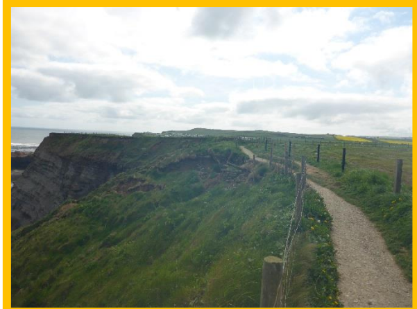
MU13/1 Recent slump encroaching coastal path (Partly Active)
