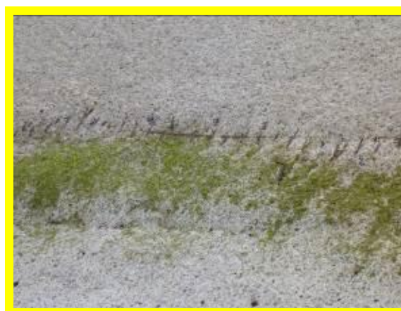
Exposed rebar (D0701C02)
