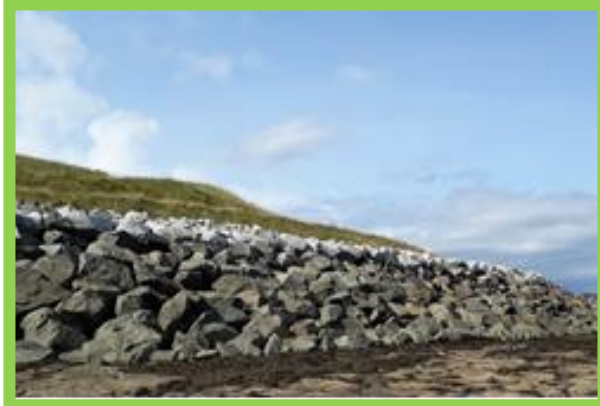
Rock revetment around debris lobe of Holbeck Hall landslide (/1304C01)
