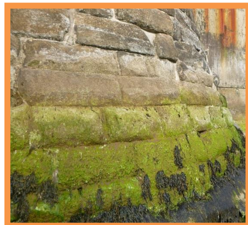
Typical defects on blockwork wall (/1003C04)
