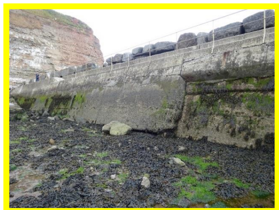
Undercutting of the inner-facing wall of North Breakwater. Seaward end (left) and landward end (right) (/0402C01)
