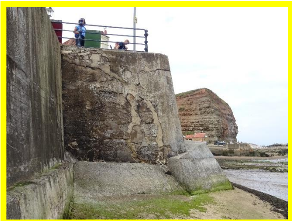
Abrasion and cracking to seawall face and crest at interface between different wall sections (/0403C05)
