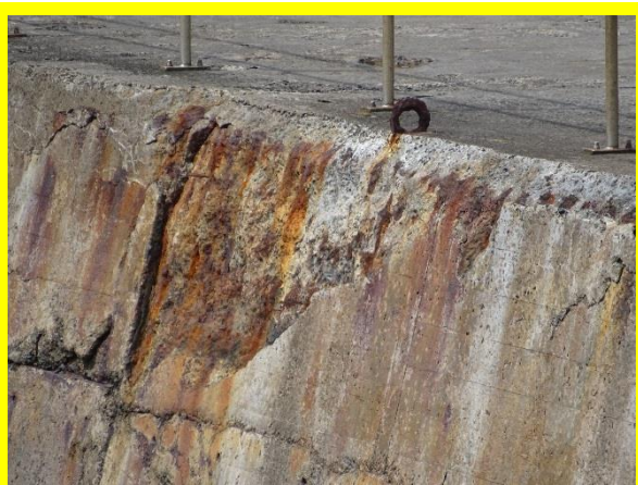
Abrasion and rust-staining on inner-facing edge of North Breakwater (/0402C01)
