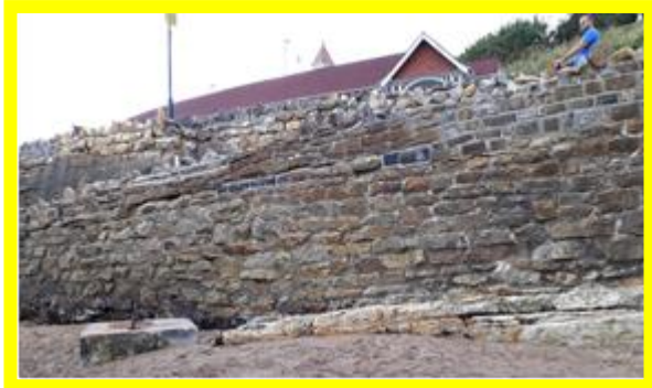
Overall fair condition of low stone wall (/1302C03)
