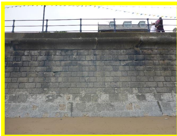
Abrasion damage and open joints in sea wall south of Cargate Hill (/1602C03)
