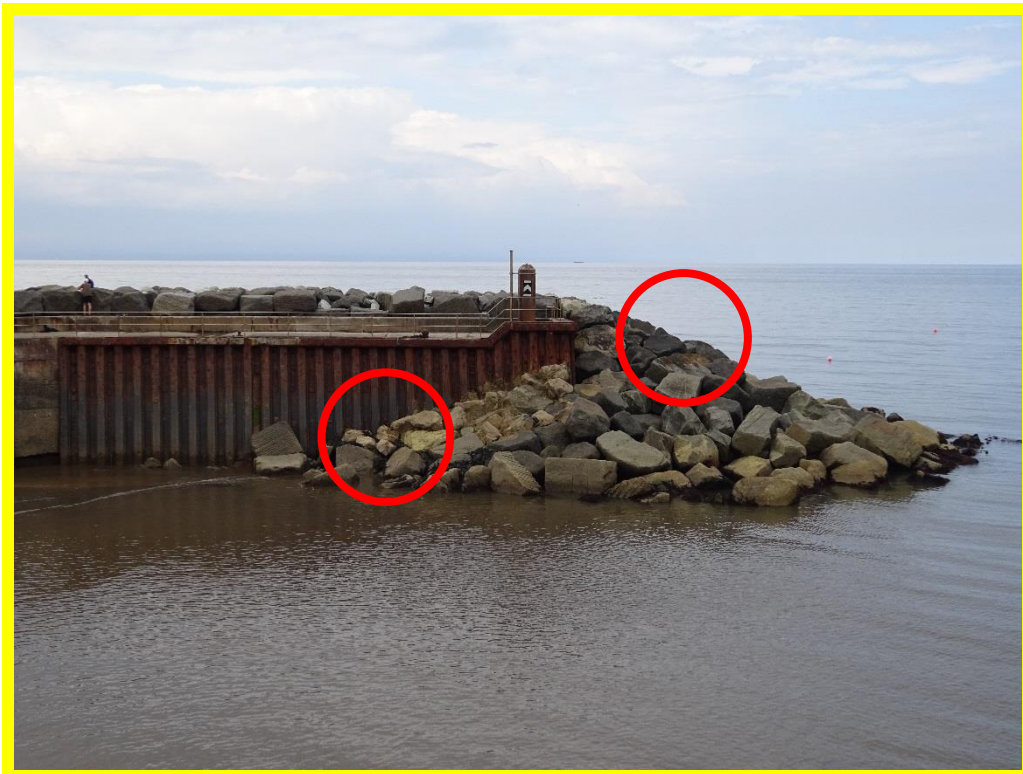
Rock armour at eastern extent of North Breakwater – possible historic movement of rocks (/0402C01)
