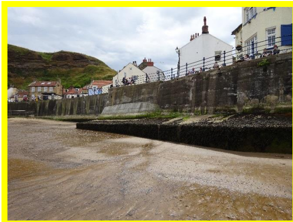
Recent toe berm addition to wall west of Cod & Lobster in Good condition, original wall in Fair condition (/0403C05)
