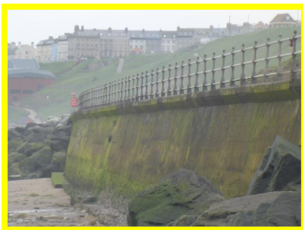
Seawall at gap in rock armour revetment (D0802C01)
