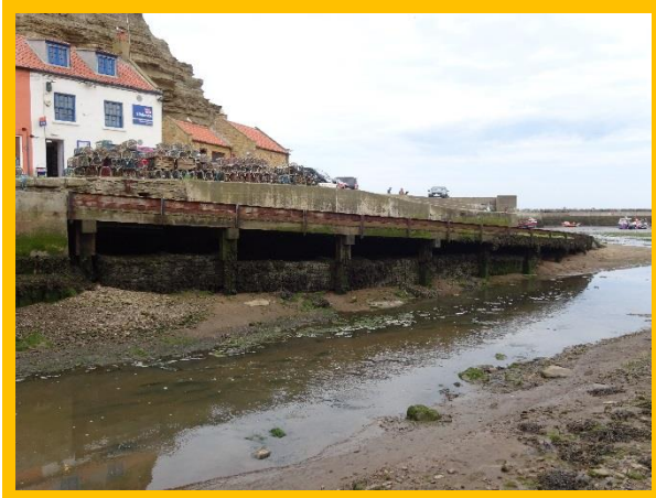
Timber slipway. Minor settlement of blocks within gabions beneath (/0402C03)
