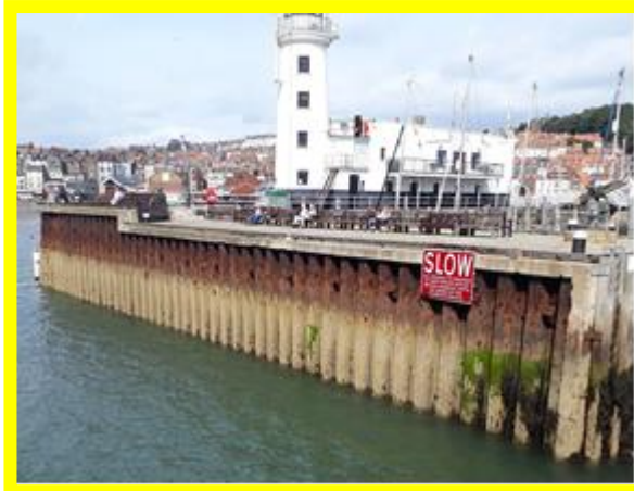
Corroded steel sheet piling (/1301C17)
