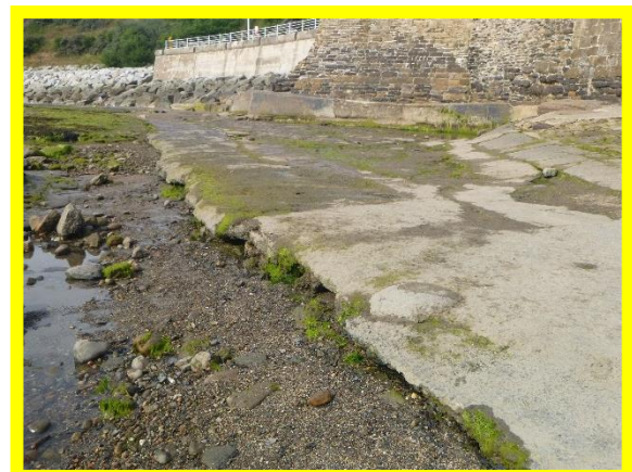
Undercutting of slipway toe and damage to previous repairs. (/1003C05)
