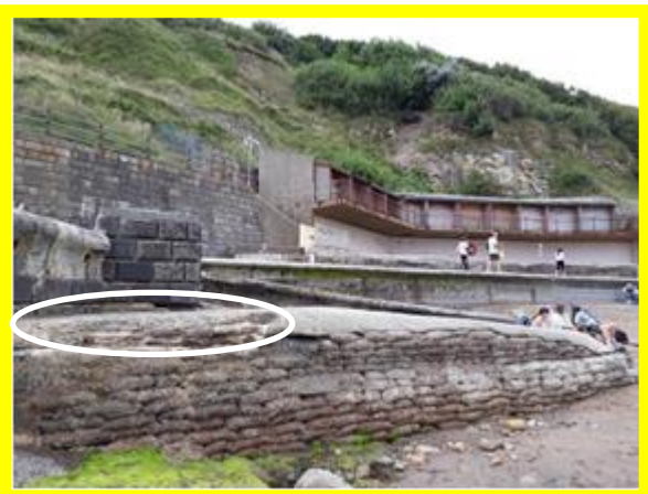
Missing area of bagwork/screed (/1302C02)
