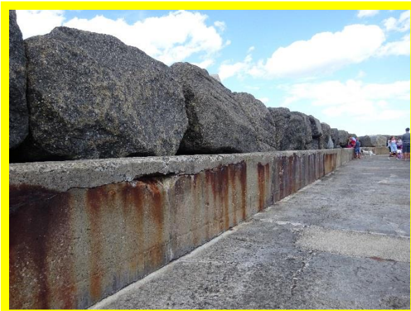
Rust staining and spalling to crest wall (/0402C01)
