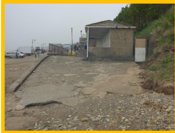
Voids in deck of rear ramp/wall at Coble Landing (/1602C01)
