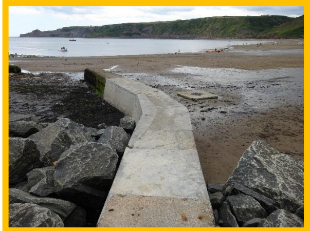
In situ poured mass concrete reinstatement of breakwater. Repair to left (/0601C02)
