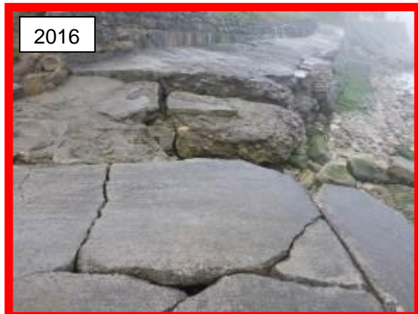
Cracked concrete at landing at beach access (/1402C06)
