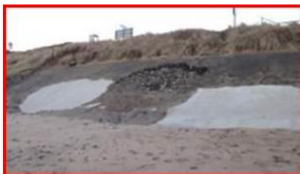
Previous storm damage and very poor condition of sloping revetment at Sandsend Road
