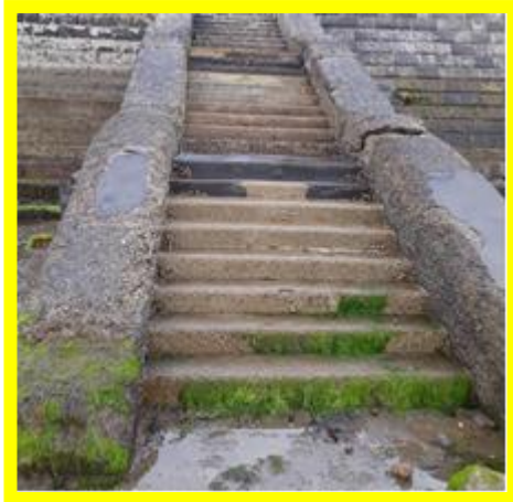
Poor condition access steps with severe corrosion to side wall toe piles (/1201C02)
