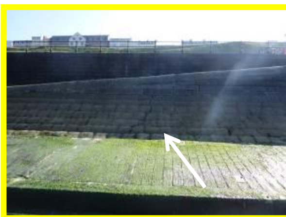
One of two notable cracks visible in wing-wall at access ramp (/1201C21)
