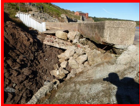
Damage to rear of structure, washout of fill material (/1402C06)
