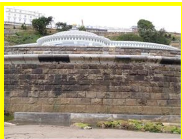
Previous repairs to wave deflector wall in front of the Sun Court & new concrete toe installed in 2017 (/1301C28)
