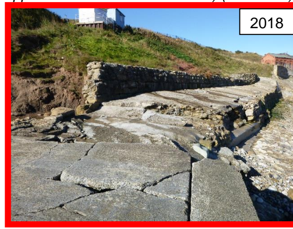
Slumping cliffs adjacent to steps leading to outflanking – southern end (/1402C04)
