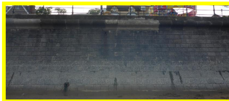
Several open joints in seawall south of Ravine Road leaking water (/1602C08)
