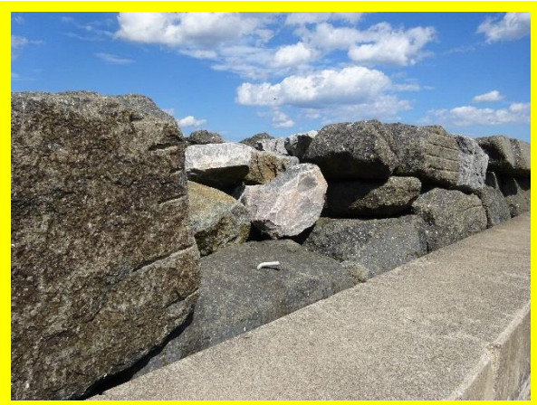
Missing crest block (30m from landward end) (/0402C01)
