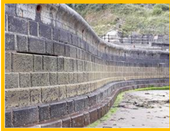
Concrete block wall with open joints and heavy abrasion (/1303C02)
