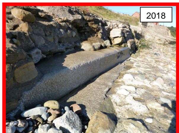
Mass concrete repair to damaged section of wall. (/1402C04)
