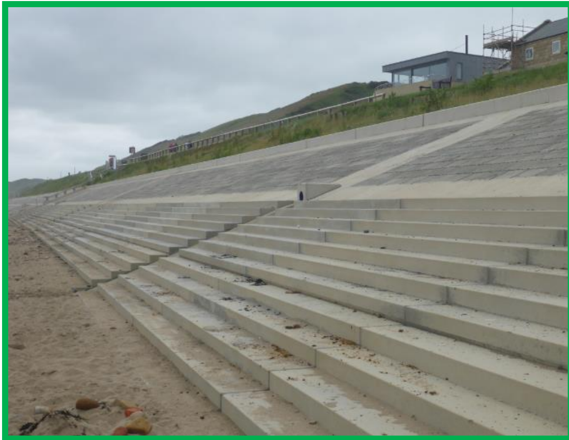
Cross section of coastal defences at Sandsend Road in 'as built' condition showing stepped pre-cast apron and upper Dycel units (D0702C02)
