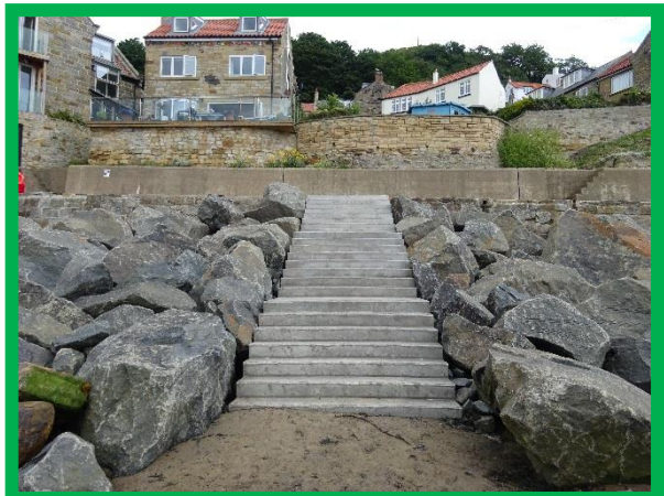
Reinforced Concrete access steps (/060C03)
