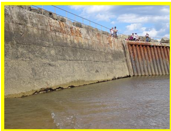
Undercutting of the inner-facing wall of North Breakwater. Seaward end (left) and landward end (right) (/0402C01)
