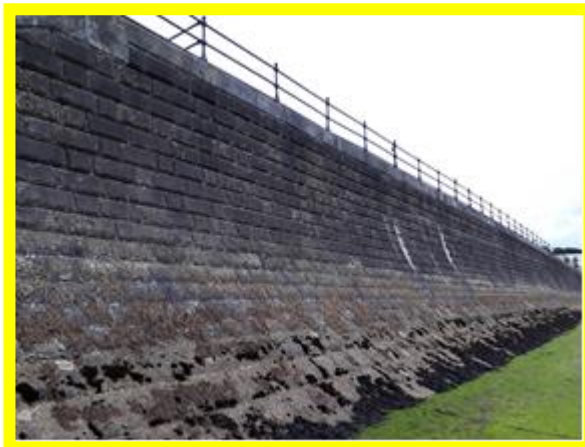
High curved-profile seawall (/1201C07)
