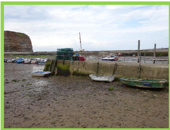
Inner harbour concrete breakwater (/0403C04)
