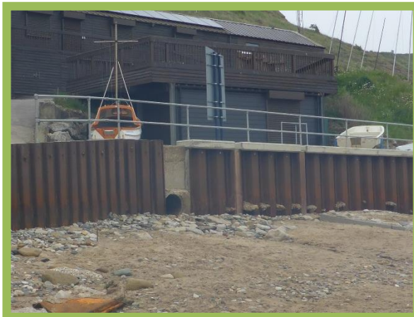
Repaired central section of steel sheet piling as observed in May 2018 (/1601C03)
