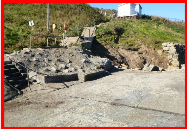
Undermining of footpath beneath 'Lucy's Shack' (/1402C04)
