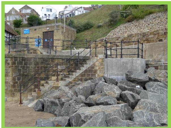
Pumping station and raised manhole chamber (/0601C07)
