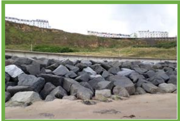
Rock armour revetment and wave return wall (/1202C03)
