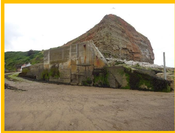
Cracks and cold joints in concrete seawall to rear of slipway (/0402C03)
