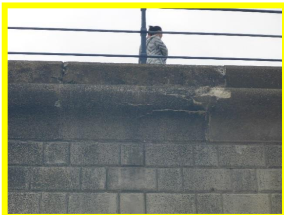
Damage to coping/wave return on seawall south of Ravine Road (/1602C08)
