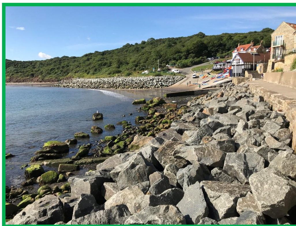
Rock armour fillet at toe of existing seawall
