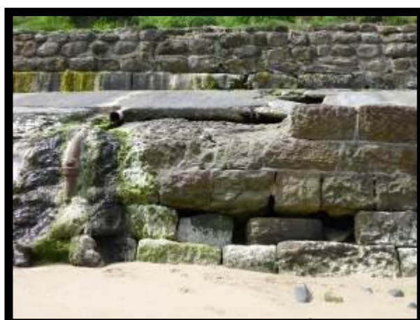
Missing blockwork in May 2015 (/1402C04)
