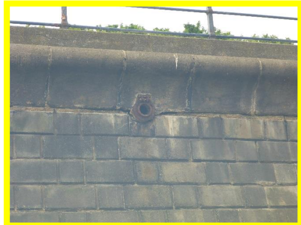
Occasional open joints with missing mortar (/1602C06)
