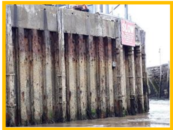
Corroded steel and cracked capping beam on seaward end of West Pier (/1301C1718)
