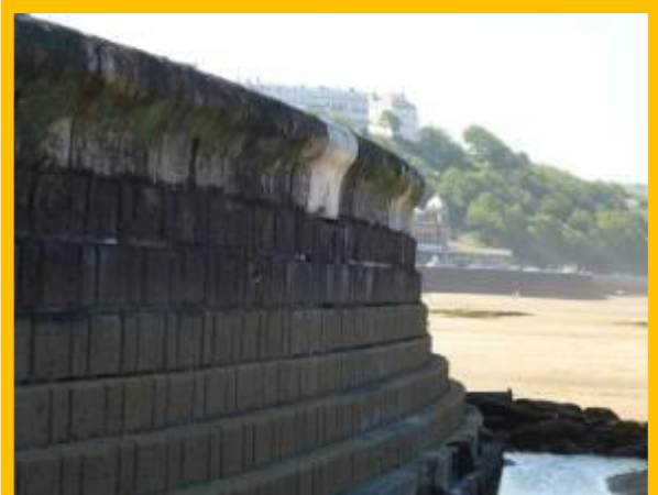
Previous repairs to wave return coping (/1303C02)
