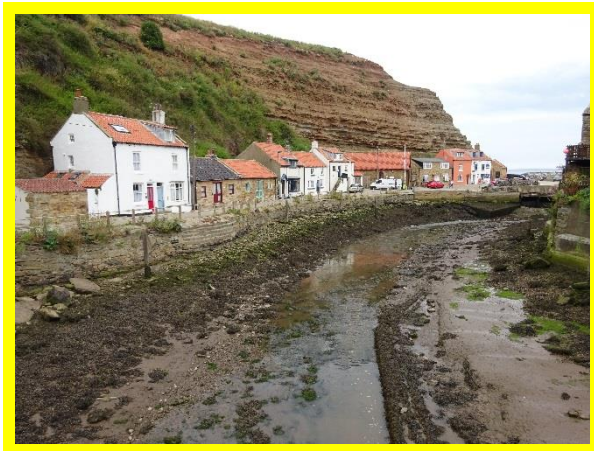
Wall on northern side of beck (missing blocks, open joints and voids) (/0402C06)
