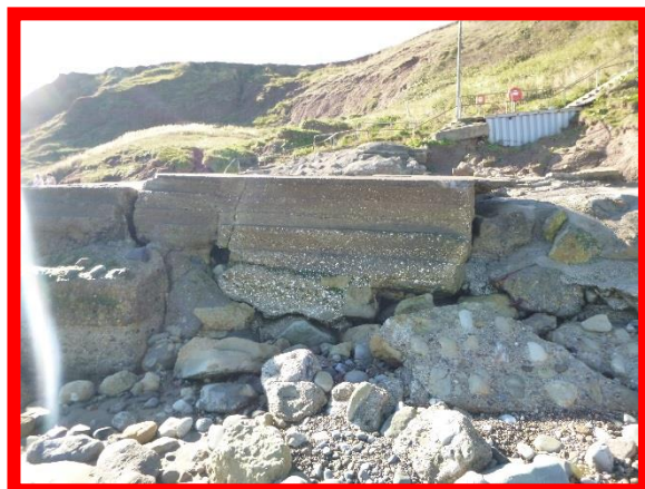
Damage to deckslab and settlement caused by washout from voids in wall face (/1402C04)
