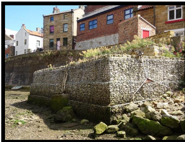
South bank: Stone-filled gabion baskets constructed in 2013 to repair collapsed wall (no asset ref)
