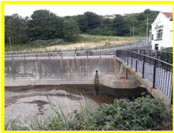
Fair condition seawall at Scalby Beck (/1201C01)
