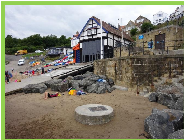
Break in rock armour fillet at pumping station (/0601C07)
