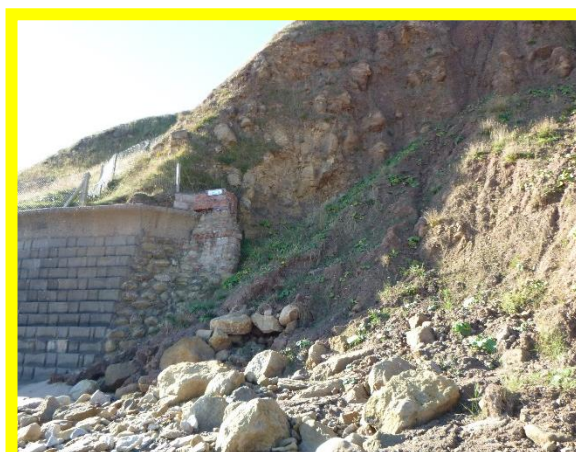
Erosion of undefended cliffs at tie-in of sea wall private sea wall (/1402C02)
