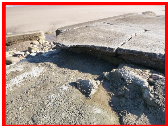
Deckslab showing signs of settlement and is significantly lifted (/1402C04)
