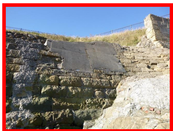
Concrete encasement at western transition (/1402C04)
