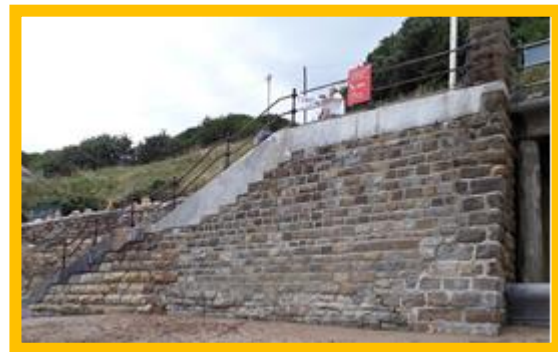
Previous repairs at southern tie-in following December 2013 storm damage (/1302C01)
