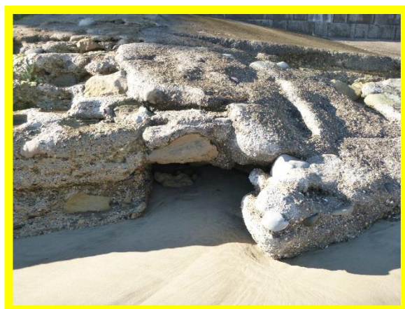
Large void in concrete apron to private sea wall (/1402C02)
