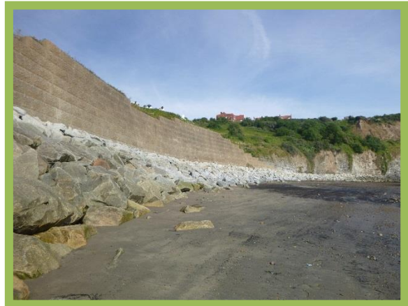
Rock revetment fronting large sea wall (/1003C01)
