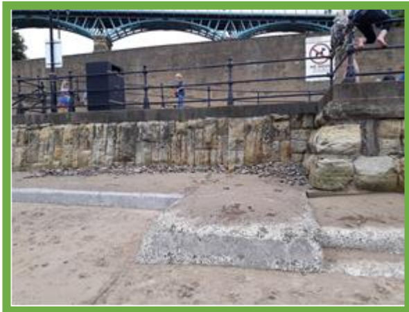
Previous repairs remain in good condition locally, but overall asset condition is fair (/1301C09)
