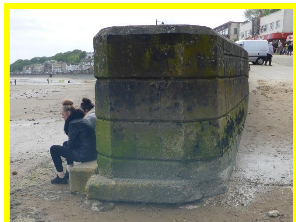
Undercutting at end of 'wing-wall' (/1602C09)
