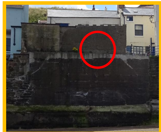
Previous repairs in lower wall. Significant crack at base of upper wall. (/0402C22)
