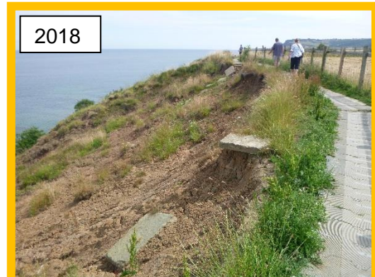
MU17/2 Undermined Cleveland Way footpath route and temporary diversion (Partly Active).
