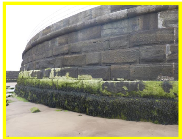
Battery Wall, with some open joints between blocks (\D0802C12)
