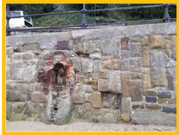
Missing blocks around Spa feature (/1301C10)
