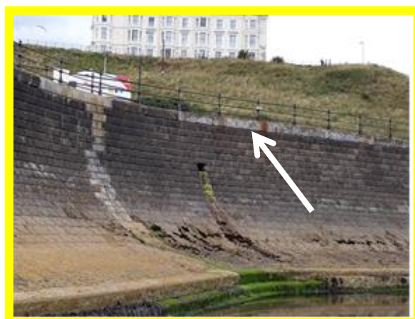
Small cracks in seawall coping adjacent to area of previous seawall repairs (/1201C21)
