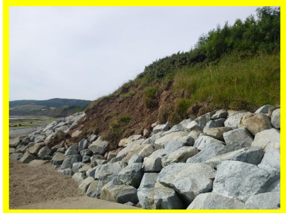
Slumping of cliffs immediately adjacent to southern end of rock armour (/1003C07)
