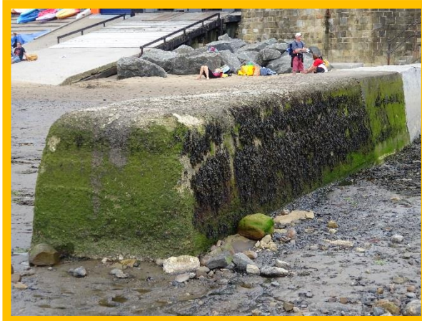
Significant abrasion of concrete. Opening of joint between wall and crest concrete – largely obscured by vegetation (/0601C02)
