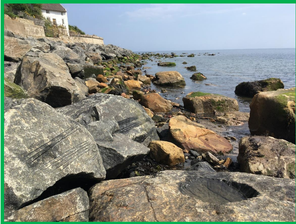
Artificial rock pool, surface scoring and natural seed rocks – ecological enhancement at the toe of the new rock armour fillet.
