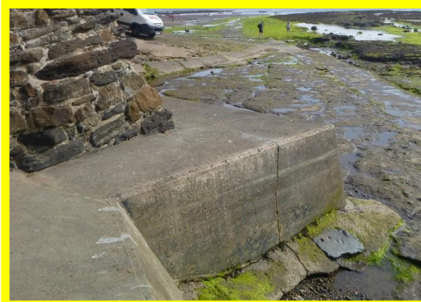
Typical defects (cracking) on toe apron (/1003C06)
