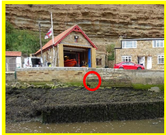
Gap at base of interface between new and older walls in front of RNLI station (/0402C06)
