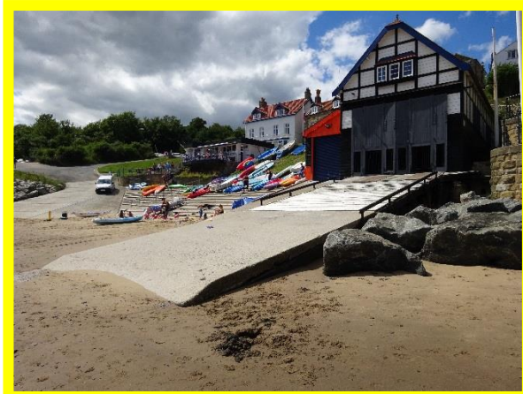
Former lifeboat slipway. Low beach levels expose previous repairs/concrete pours at the toe (/1003C04)
